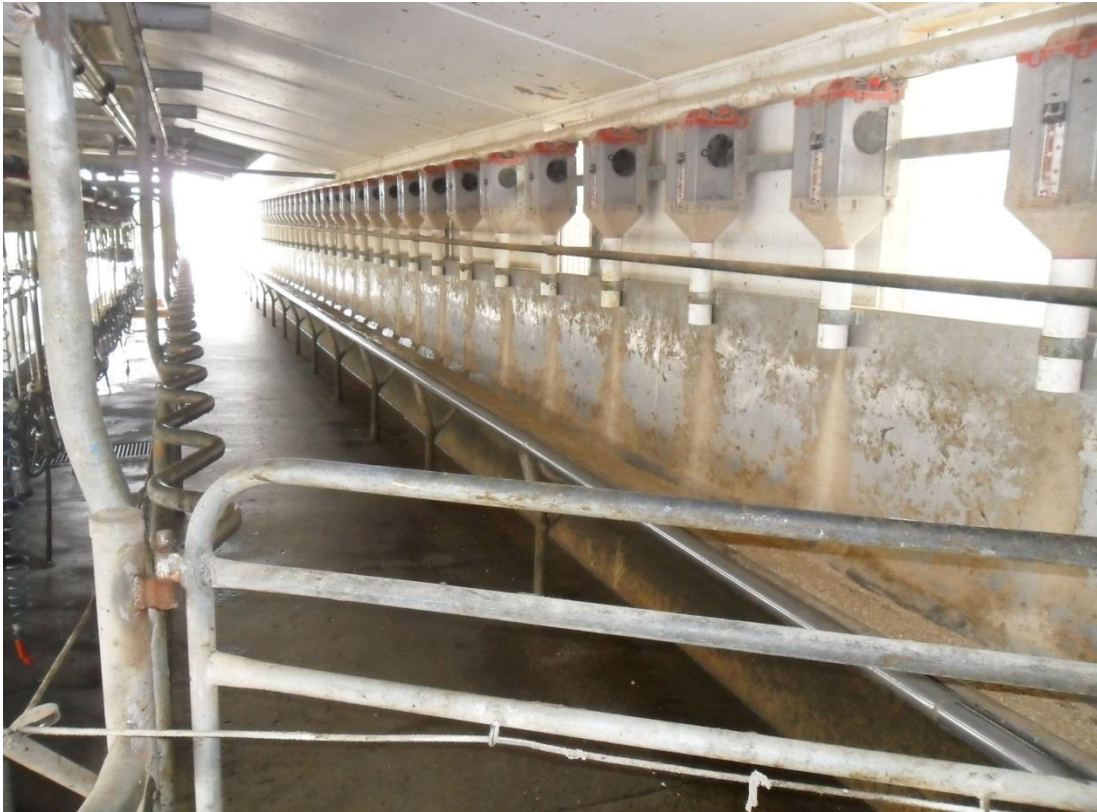
Figure 5. The empty milking shed
