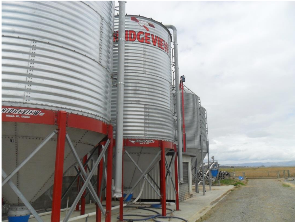
Figure 13. The feed system outside the shed
