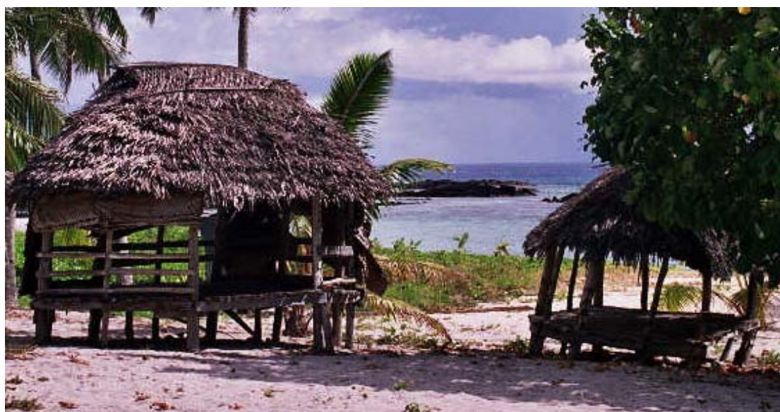
Figure 3: Dilapidated Beach Fale
